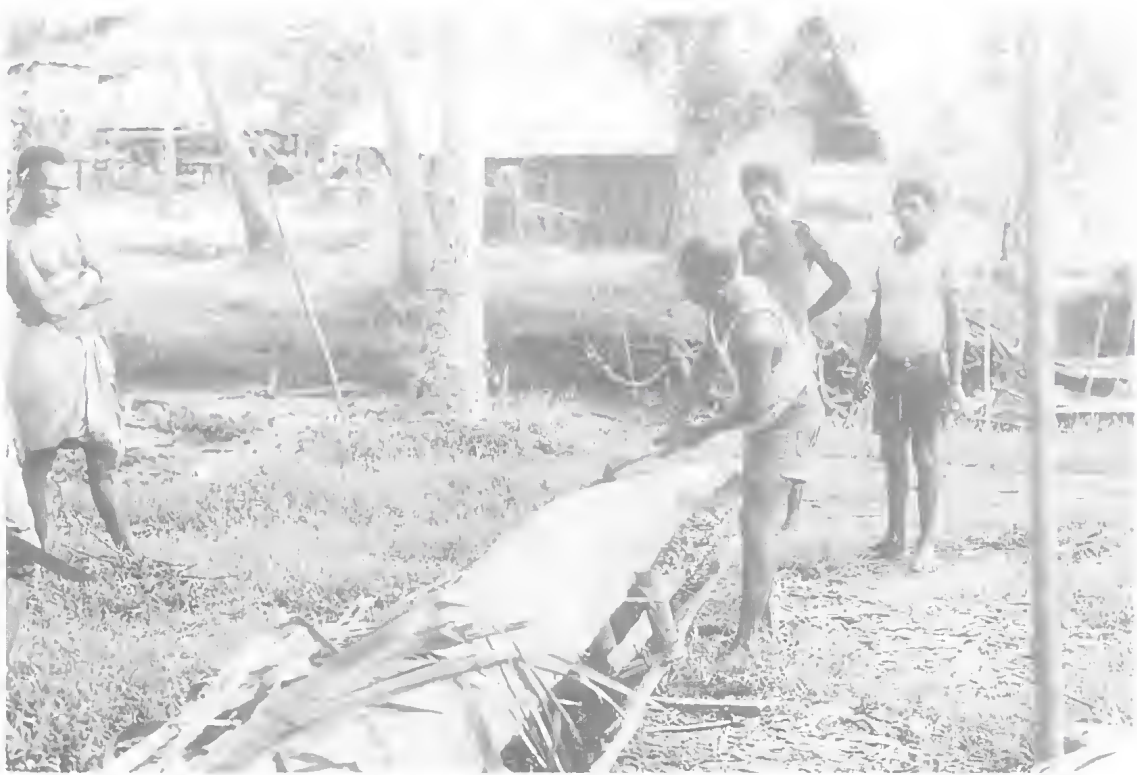
FIG. 53. Shaping and cleaning the outside of a canoe hull using a metal axe, Madame village, Fly estuary.
